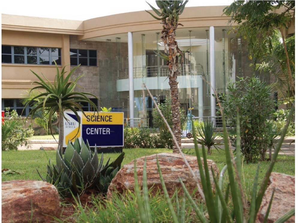
USIU-Africa, Science Centre Building.
